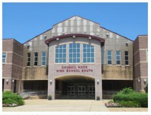
The prefinished aluminum-skinned metal panels finish greatly diminished over the past year. The panels should be considered for refinishing or replacement. The panels at the rising walls above the Auditorium are in a similar condition and should be included as a part of the project.
